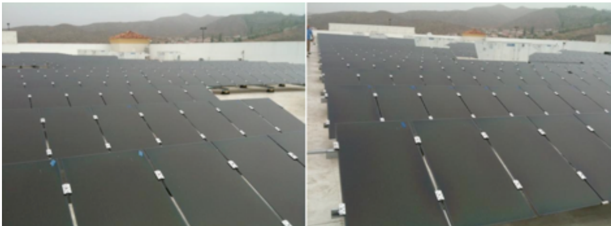
Fig. 2: All bad modules were identified and marked with blue masking tape in the right hand corner.
